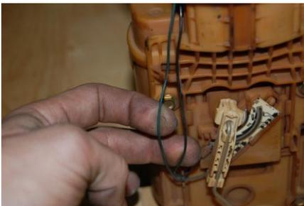
3. Once you have confirmed that the connections have been made correctly you can begin to heat shrink them. The butt connectors have heat shrink ends, simply heat the ends slightly with a heat gun until they seal completely around the wire.
